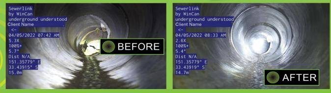
SureSearch uses QuickView cameras to check drains after clearing pipes. Our Jet Vac Drain Cleaning technicians have experience in dealing with all sorts of drainage projects issues, from heavy cleaning of storm water culverts and systems to mass infestation of tree roots in sewer networks.
